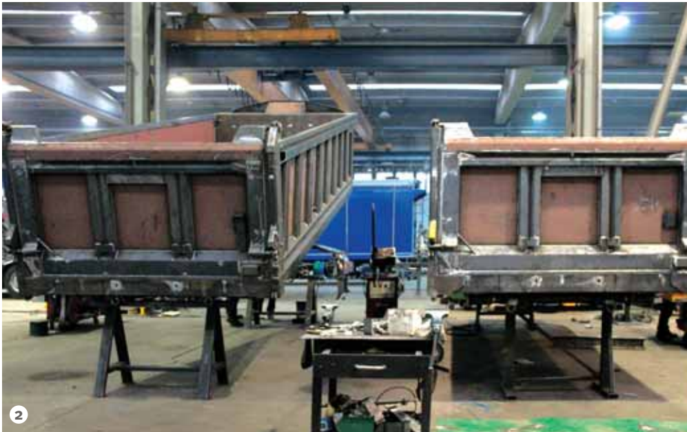
Figure 2: The container building phase.
